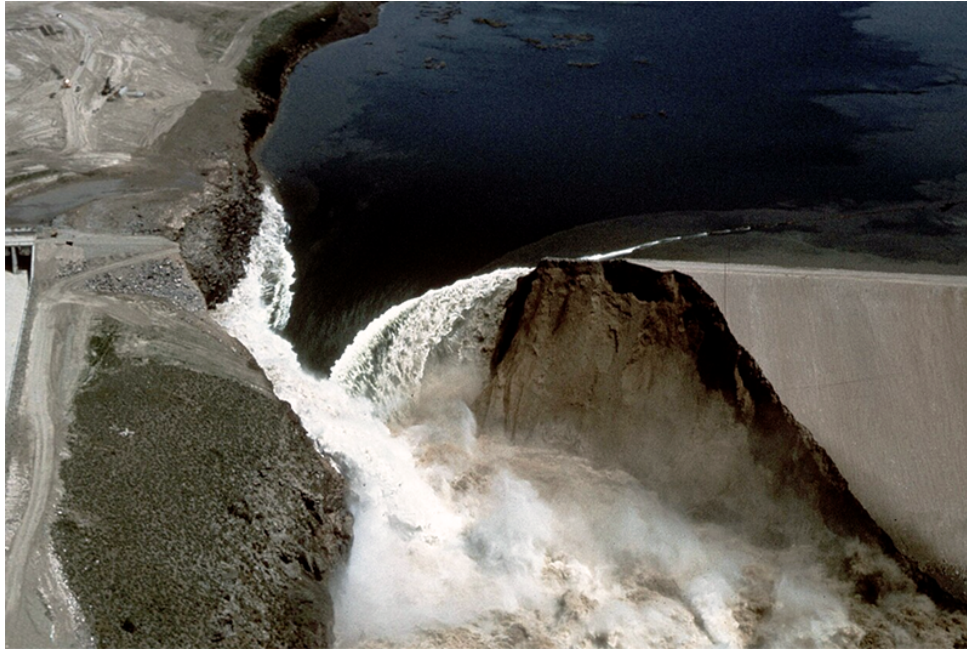
Fig. 1 Failure of Teton Dam, on the Teton river, in eastern Idaho, on June 5, 1976, possibly a rare instance of a mixed kinematic-dynamic wave.
